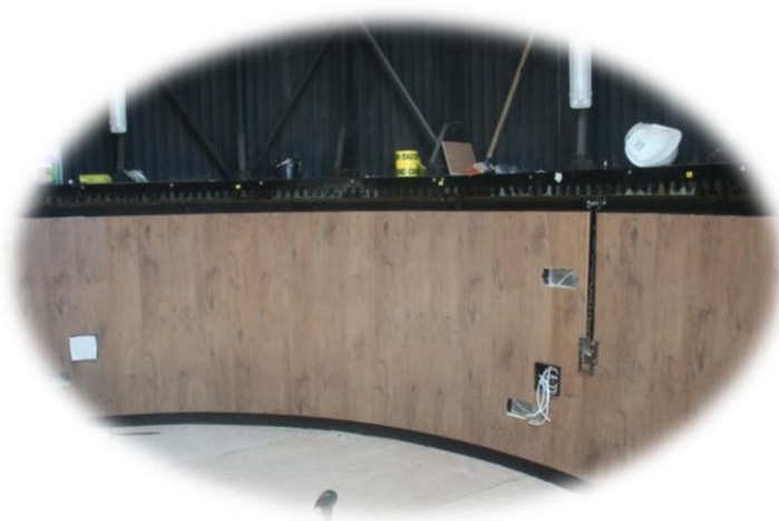
Hampshire AG 24" dome: New floor laid and refurb nears completion
