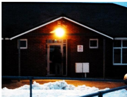
An example of glare from the Pavilion security light hiding a man at the door.
